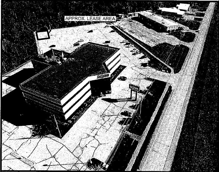
C SITE OVERVIEW (LOOKING NORTH)
